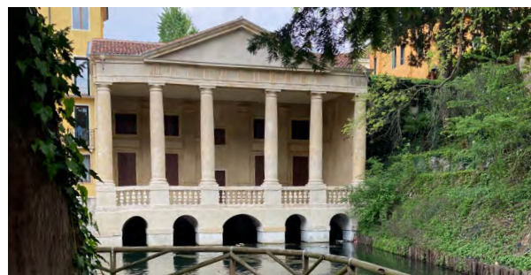
Figure 06 | View of Loggia Valmarana from Seriola watercourse.
