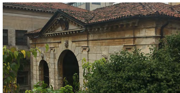
Figure 07 | View of Loggia Longhena from Seriola Fair pavillon rooftop.
